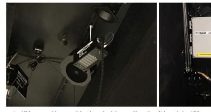
An IFS control box and fog head with an effect fan (L) and the IFS pump station (R)
